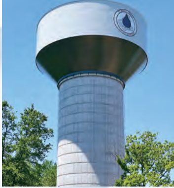
The new 2-million-gallon South Ola Water Tank is the largest above ground storage within the HCWA system.
