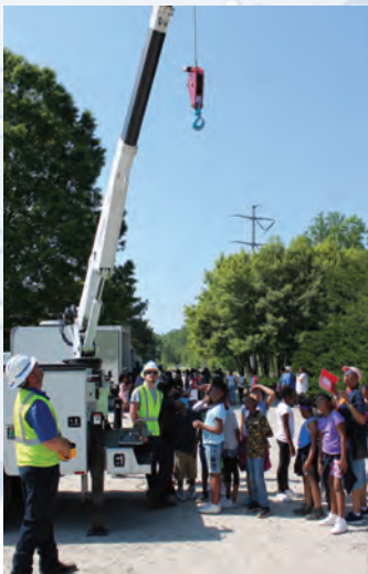
HCWA Maintenance Mechanics Chris Kuhn (far left) and Robert Sims explain the use of this truck and crane for maintenance of the utility's infrastructure.
